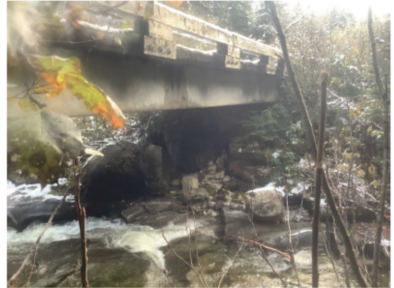
Right Bank Abutment when facing downstream
