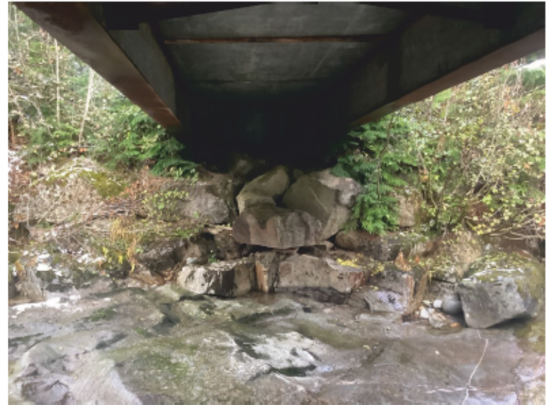
Left Bank Abutment when facing downstream
